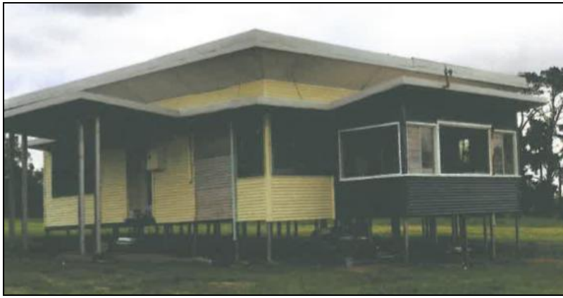
House transported to 1348 Arthur River Road – Dinninup
