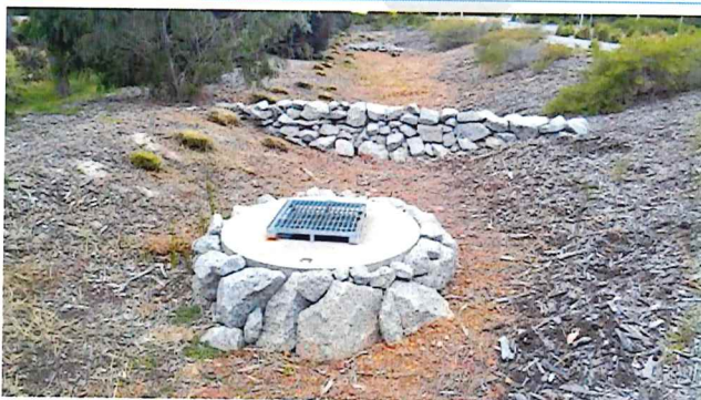
Figure 19 – Example – storm-water management – open drain
