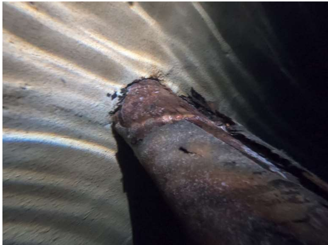
Original pipe penetrations – NO LEAKS
