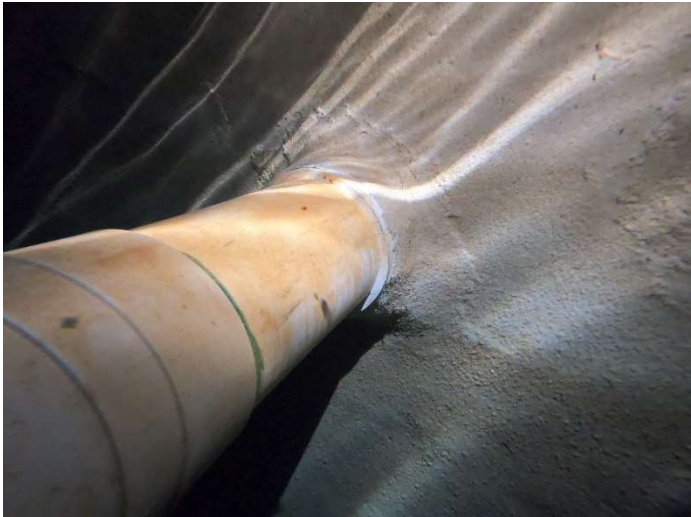
Balance tank penetrations – NO LEAKS
