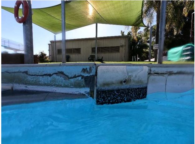
Capping screed cracking
