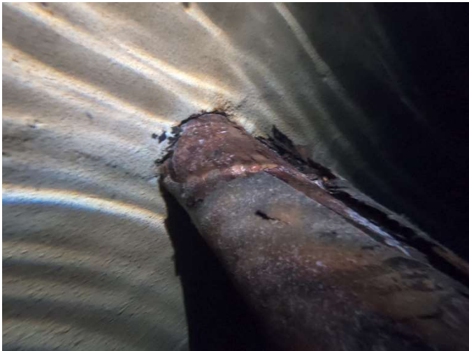
Original pipe penetrations – NO LEAKS
