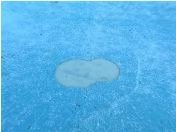
Capping screed cracking
