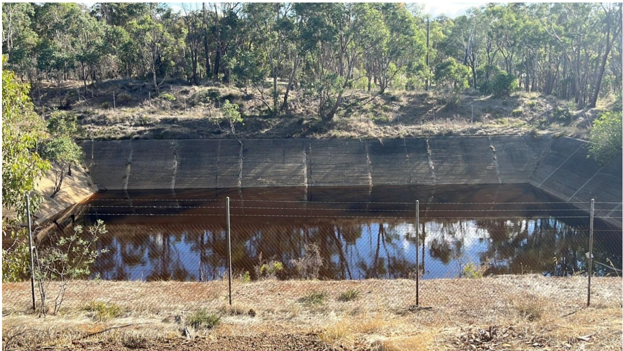
Railway Reserve dam
