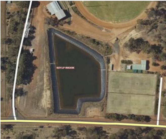
Aerial view of dam
