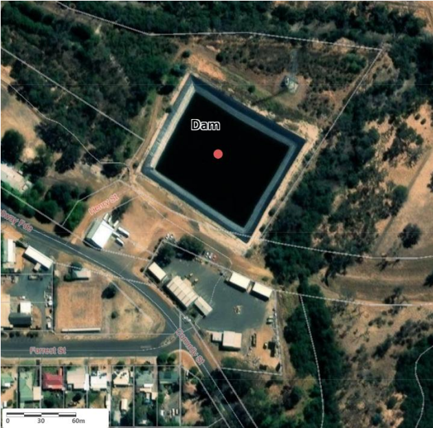
Aerial of dam
