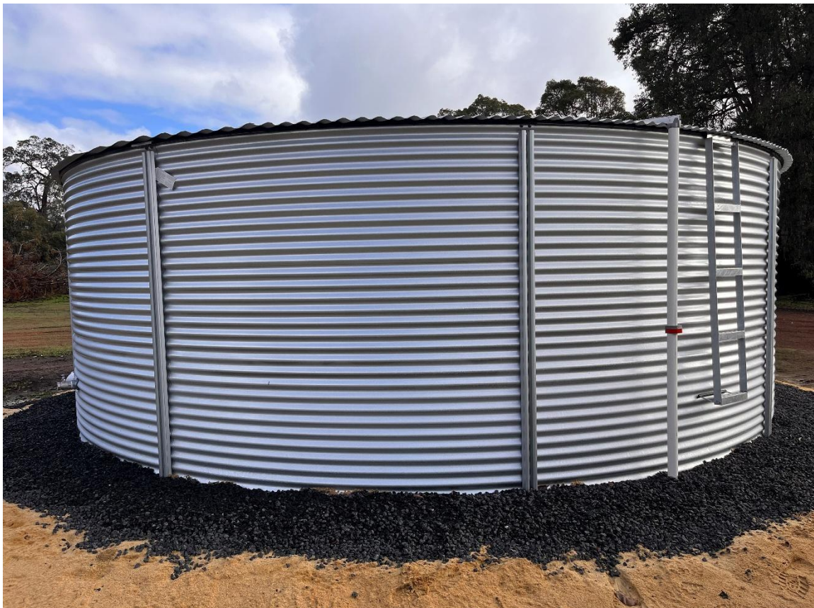
Wilga Hall Fire Emergency Tank
