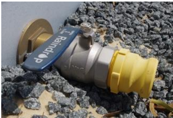
Figure 1: Standard tank camlock fittings
