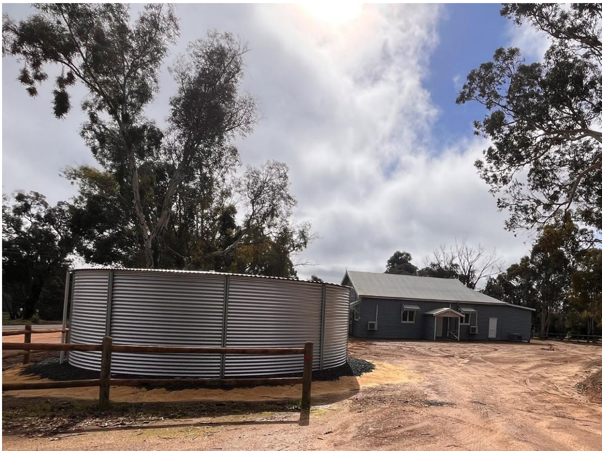
Mayanup Hall Fire Emergency Tank
