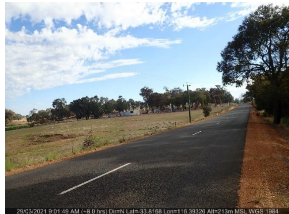
Photo ID: Photo 2 Looking at the bitumen road that services the development site.
