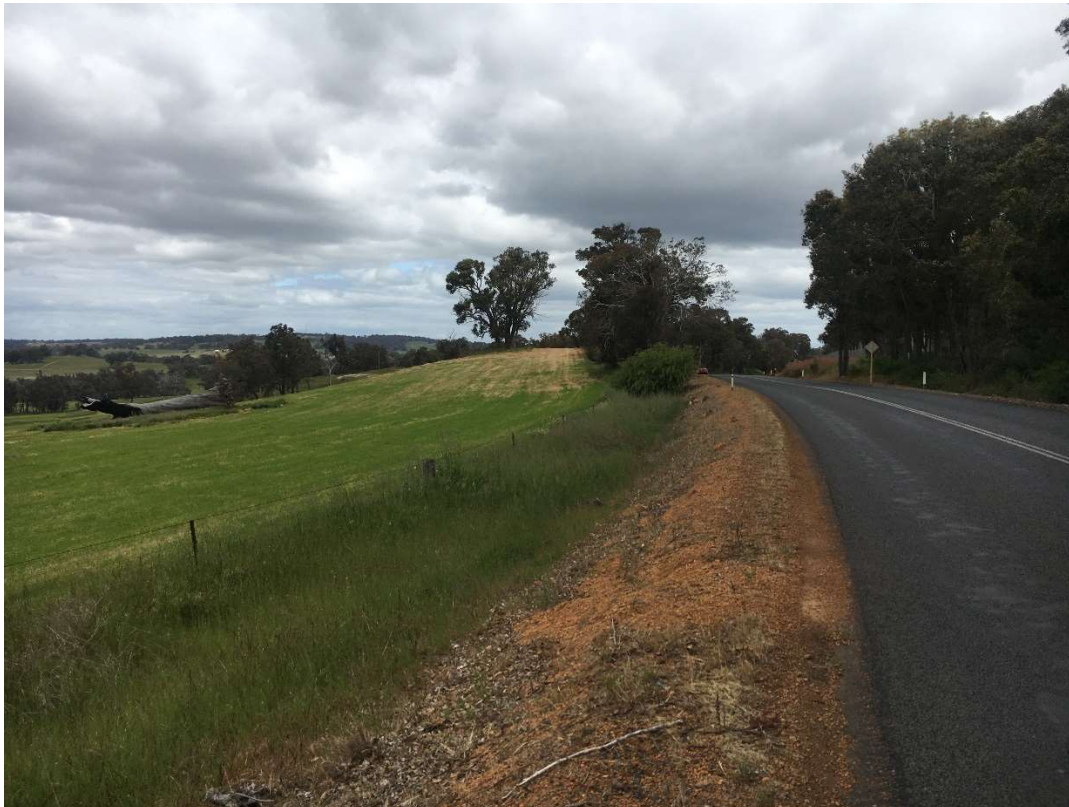
Photo 2: Road 1 View Looking from North to Intersection
