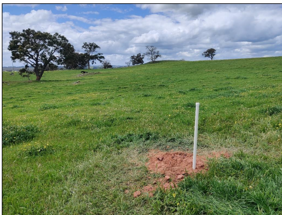
Figure 2: Installation of monitoring wells
