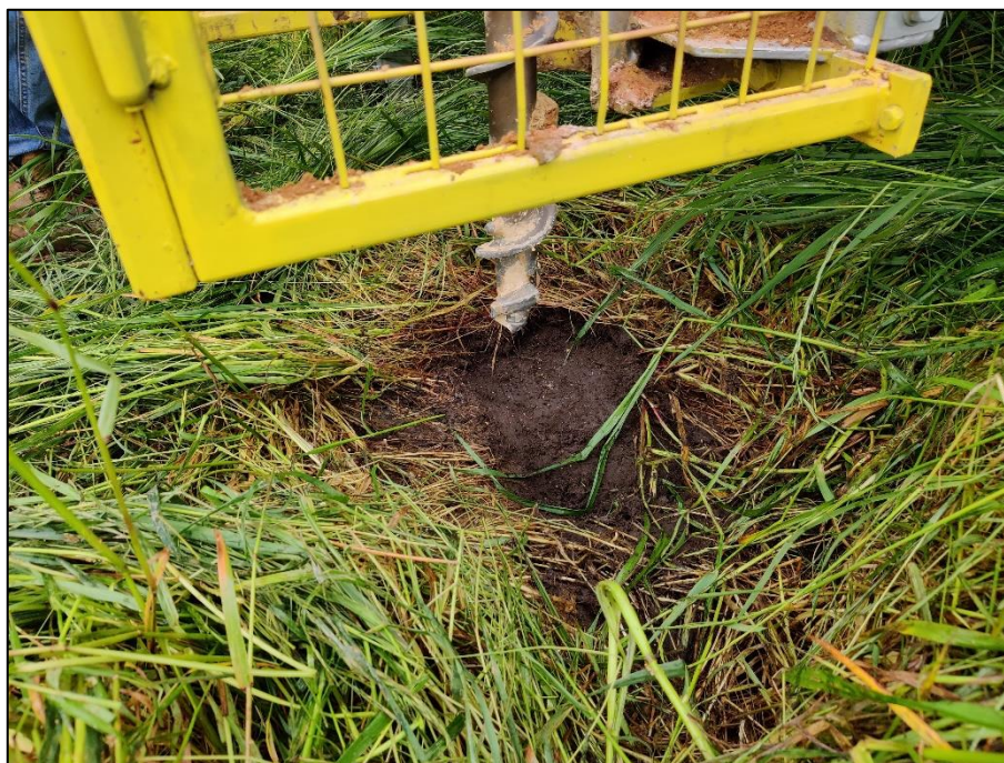
Figure 3: Tip of drill rig auger
