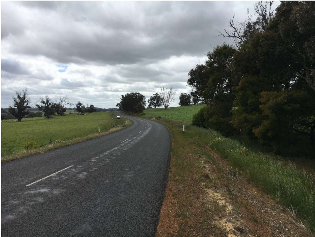
Photo 3: Road 2 View Looking East
