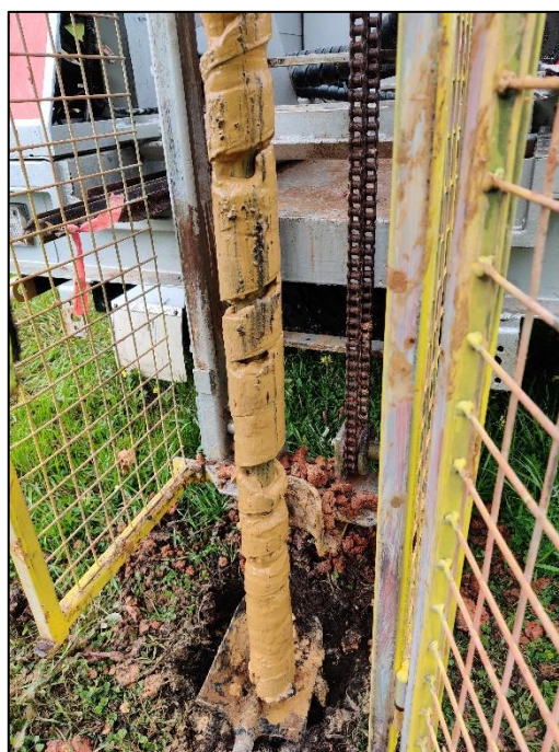
Figure 6: Drill rig used for boreholes
