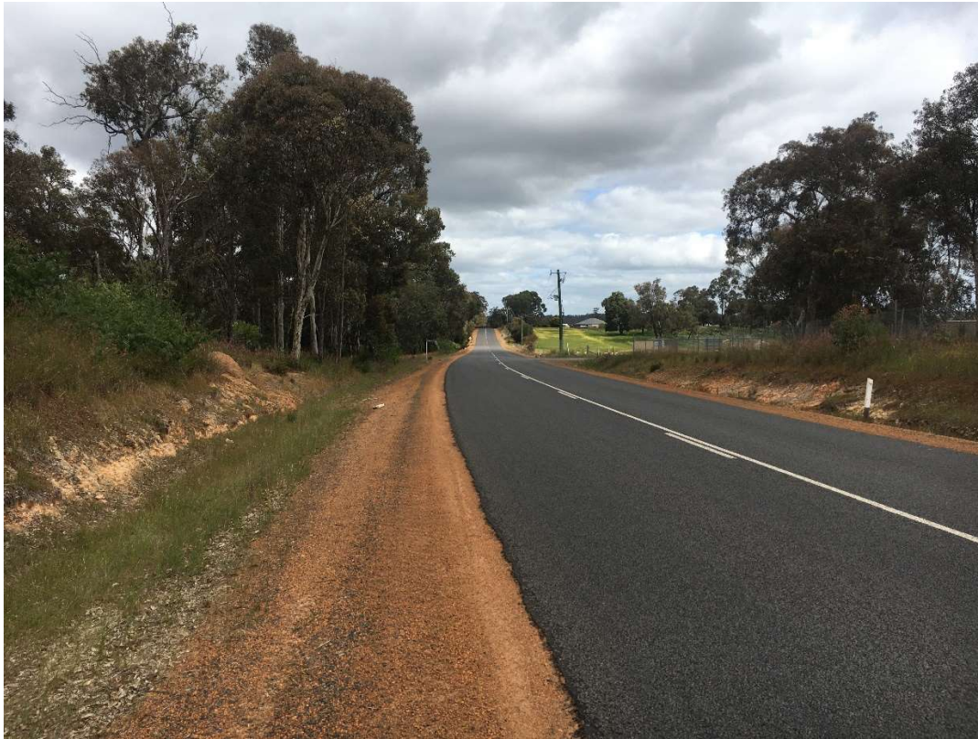
Photo 1: Road 1 View Looking South
