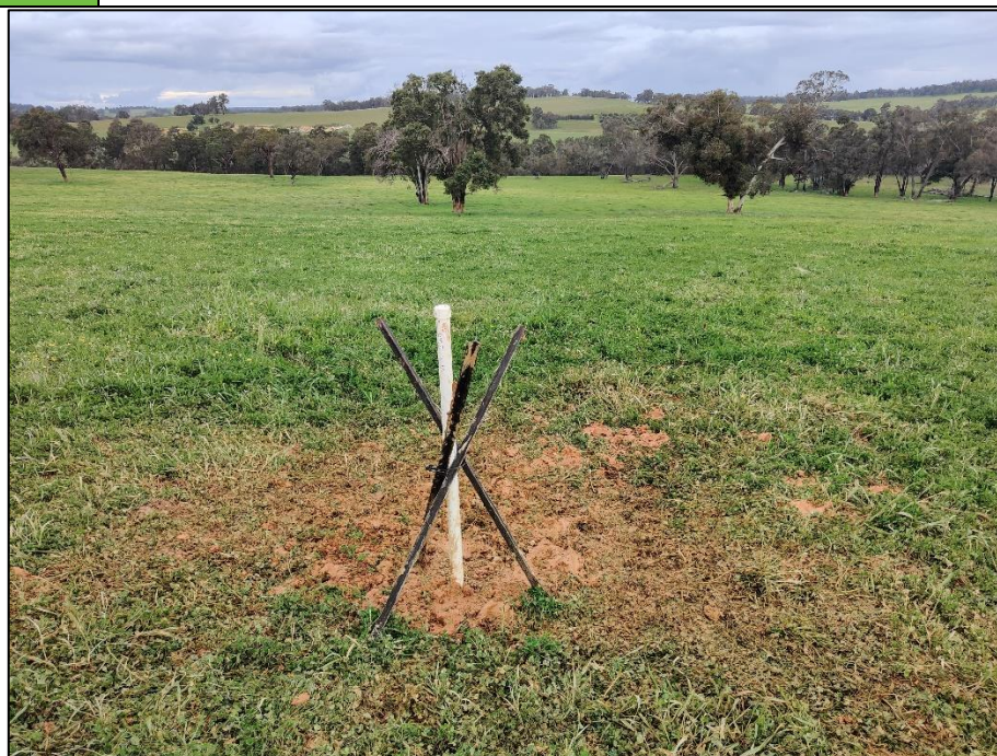
Figure 5: Installation of monitoring wells
