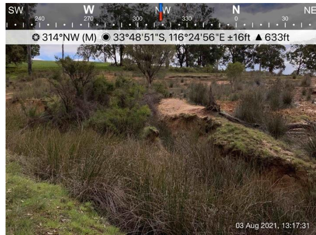
Photo 6: The lower reaches of the eastern creek line, characterized by deep eroded creek banks and trickle flow towards Blackwood River.
