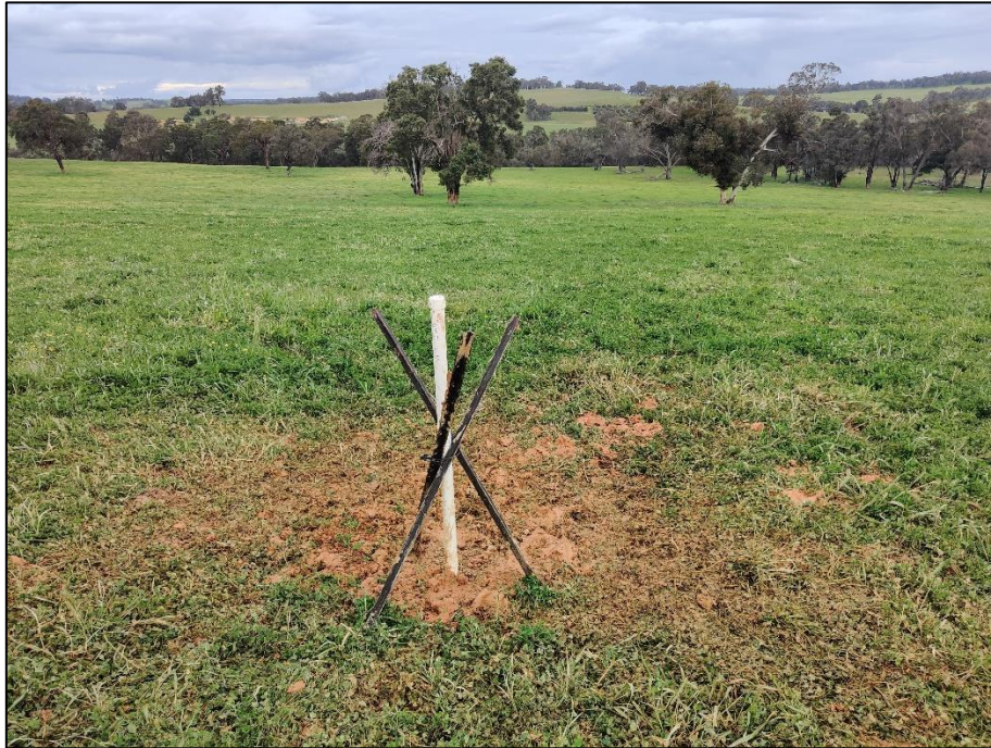
Figure 5: Installation of monitoring wells
