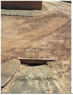
Bridge Street Between Post Office and Medical Centre Scope: Remove paving and replaced with concrete. Replace kerbing near the Medical Centre.
