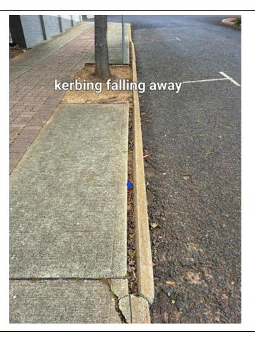
Cailes Street crn. Forrest Street Scope: Remove broken concrete slabs and replace.
