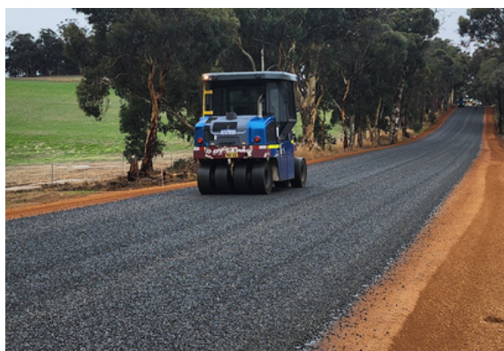
Left: works being completed on the Boyup Brook–Arthur River Road.
