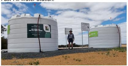
With interchangeable fittings allowing for all vehicle types, the two 50,000 litre water tanks have the ability to fill six vehicles at the same time, with a recent exercise fillina a 2000 litre fire truck in just 90 seconds. The secret to the success of the project is the overall design. The site of the tanks is sloped to ensure clear vision, easy access for all vehicle types and has a dam dedicated to filling the tanks, ensuring they stay filled and ready to use.
